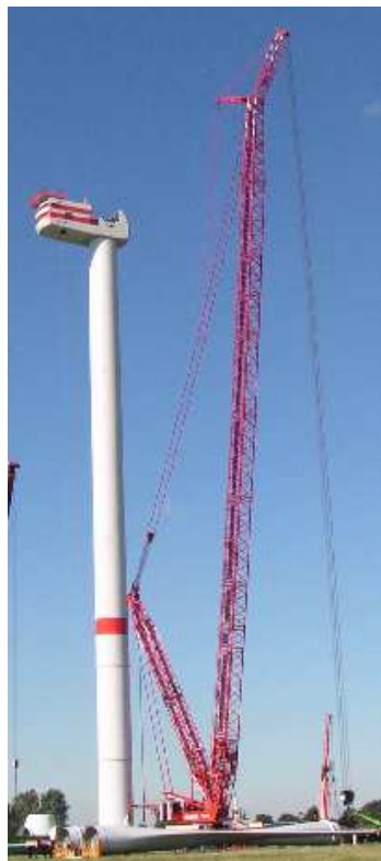
Fig. 1: REpower 5M in the erection phase
