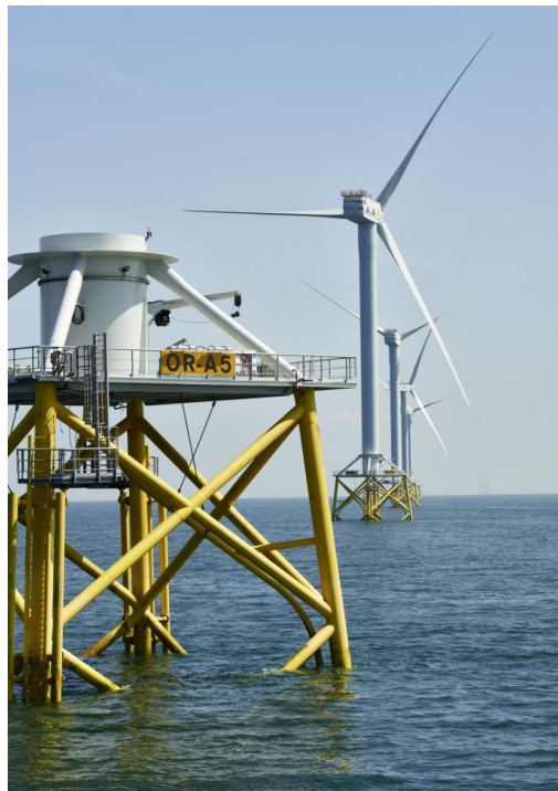
Figure 1: Senvion 5M turbine on jacket (Ormonde project)
